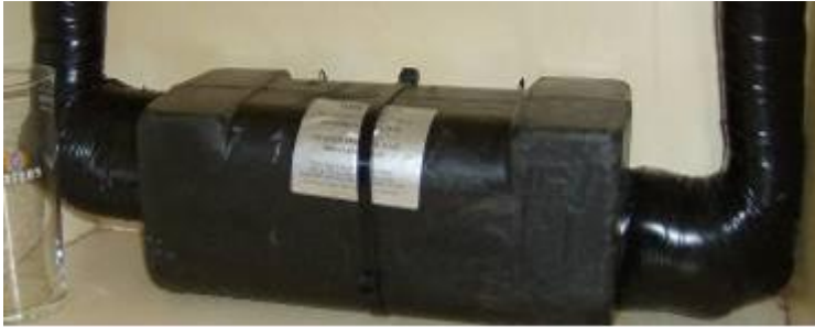
Example of correctly insulated pod
